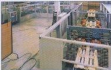
A view of the complete installation
